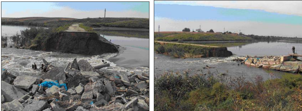
Figures 6 and 7 – Broken damn on Lake Buftea (September 2005)
